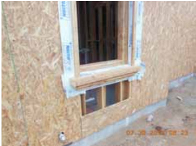
1. Exterior recessed framing condition
